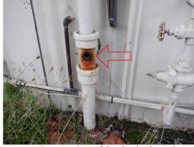
Plumbing: Some sections of the pluming have signs of rust and holes
