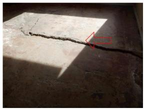
Interior Foundation unit 3121: Settlement type cracks observed on the slab
